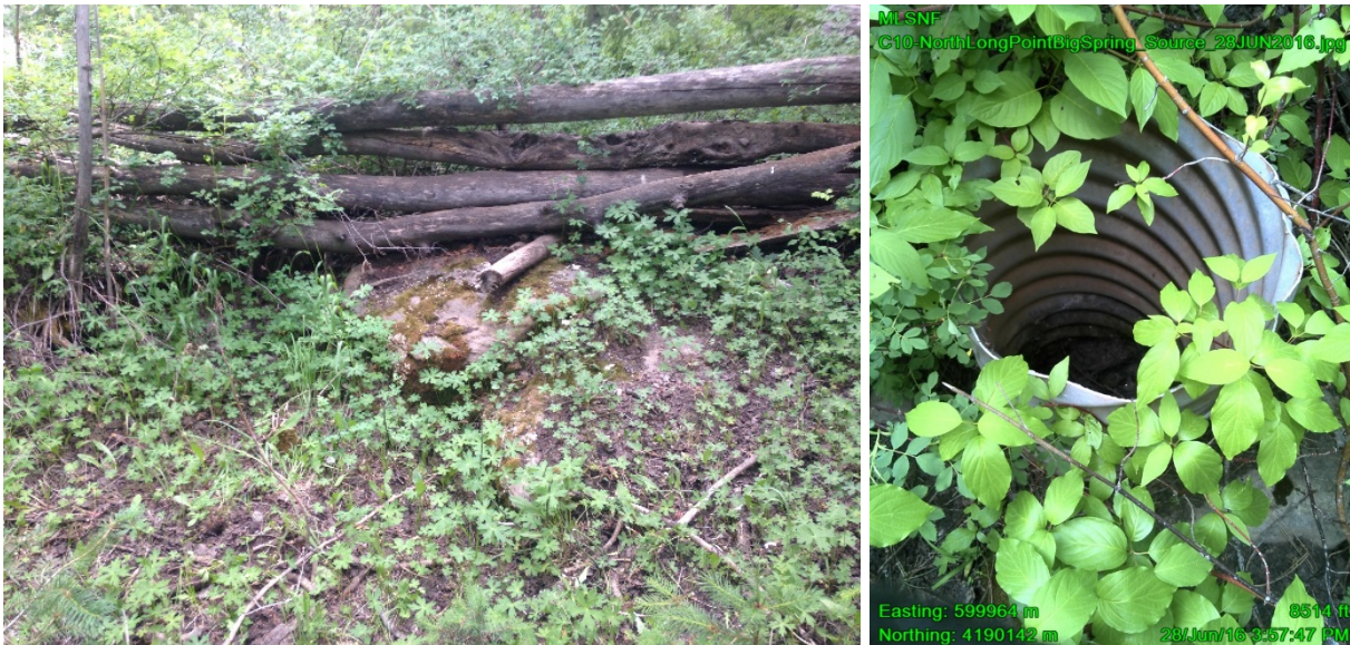
Photograph Set 7 (June 28, 2016) – Source enclosure (left) and developed source (right) at North Long Point/Big Spring (right). Right photograph is georeferenced and indicated in the field map (Figure 1).
