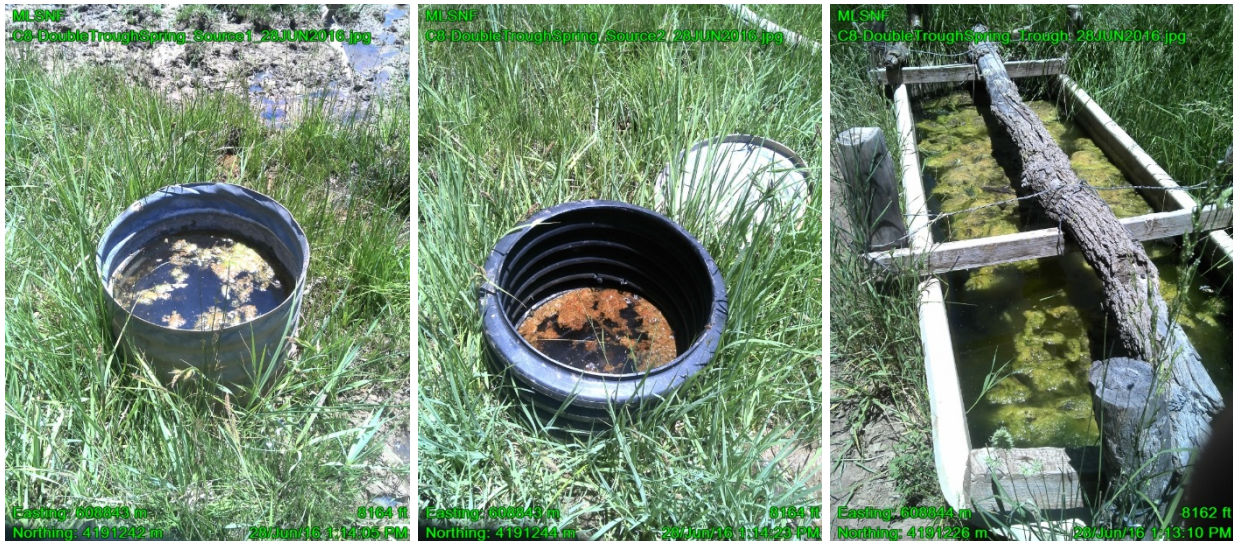
Photograph Set 4 (June 28, 2016) – Spring sources were developed with culverts (left, middle) and trough (right) at C8-Double Trough Spring. Photographs are georeferenced and indicated in the field map (Figure 1).
