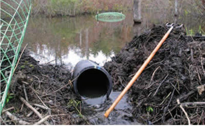
ABOVE: Pond Leveler being installed. BELOW: Preparing the pipe using a circular saw.
