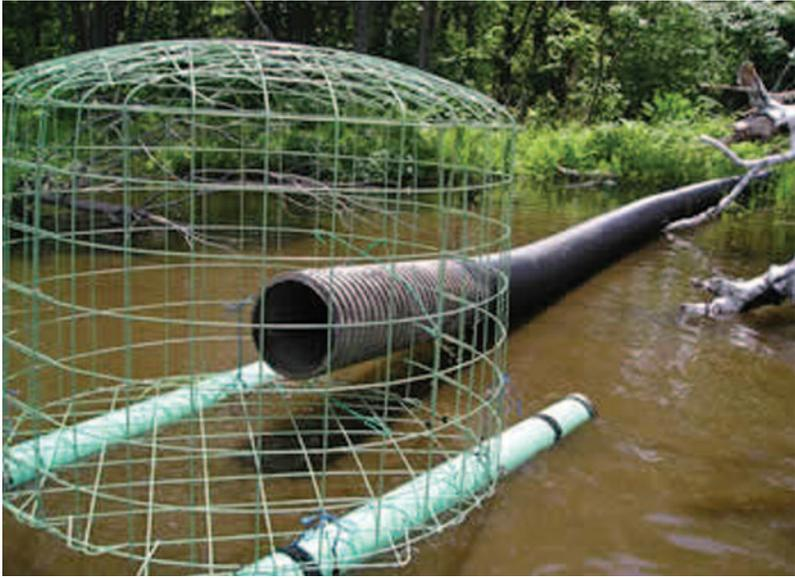
Pond Leveler intake cage with pipe. Note that the intake cage is being floated into place on two plastic floats made from capped sewer pipes. This trick, devised by Mike Callahan of BeaverSolutions.com, is very helpful for deeper ponds.
