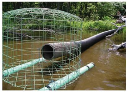
Pond Leveler intake cage with pipe. Note that the intake cage is being floated into place on two plastic floats made from capped sewer pipes. This trick, devised by Mike Callahan of BeaverSolutions.com, is very helpful for deeper ponds.
