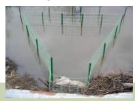
the culvert remains free of obstruction. Consider the average, as well as maximum flows expected at the site when determining the appropriate action.
