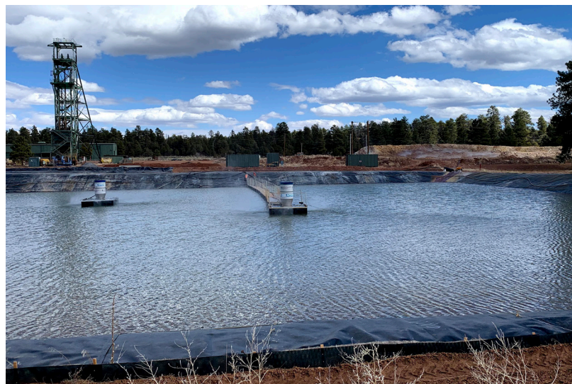
Enhanced evaporators at work in the middle of the evaporation pond at Canyon Mine on March 7, 2020. AMBER REIMONDO
