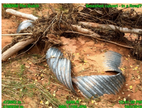
Fig. 103 Smashed culvert; in a flood?
