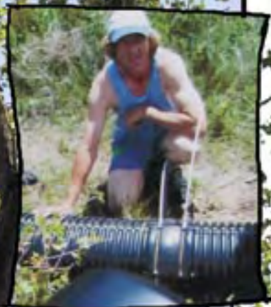
FIG. 2-B Volunteer Steve Reddy is using the right ties!
