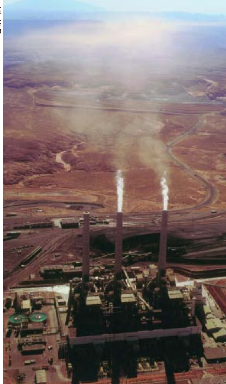
Mohave Generating Station.
