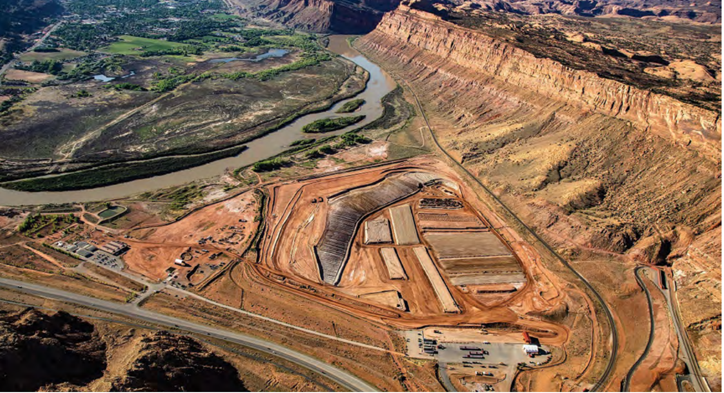
Atlas Mill site. U.S. DEPARTMENT OF ENERGY
